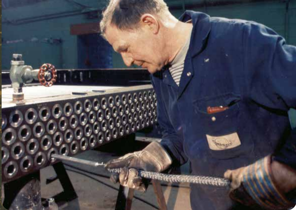
Air-cooler for Shell Oil, Nigeria, fitted with hiTRAN Matrix Elements in less than 3 hours.
