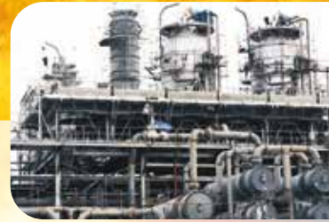
High pour-point lube-stock coolers. Designed for minimum size and high wall temperature to overcome pour-point effects. Design & fabrication: Heat Exchangers International, Australia. Contractor: LG Industries Courtesy: Thai Petrochemicals
