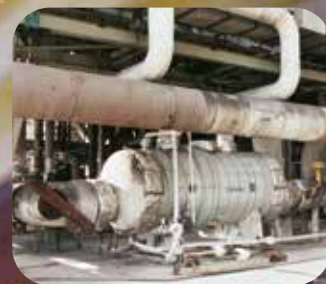
Paraxylene Feed Vaporiser/Reactor Effluent Interchanger. Increased duty to overcome capacity and space limitation. Courtesy: Huntsman Chemicals (ICI UK)
