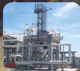
Methanol Synthesis tube-cooled converter. Higher duty retrofit. Location: Laverton, Victoria, Australia Courtesy: Coogee Energy Pty Ltd
