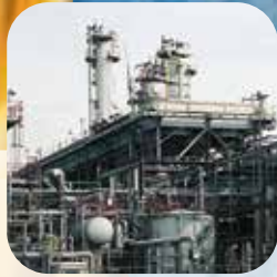
Heavy wax distillate cooling (atmospheric residue). Higher duty to meet column control need. Installed: 1992 Location: Grangemouth, Scotland. Courtesy: BP Oil, UK
