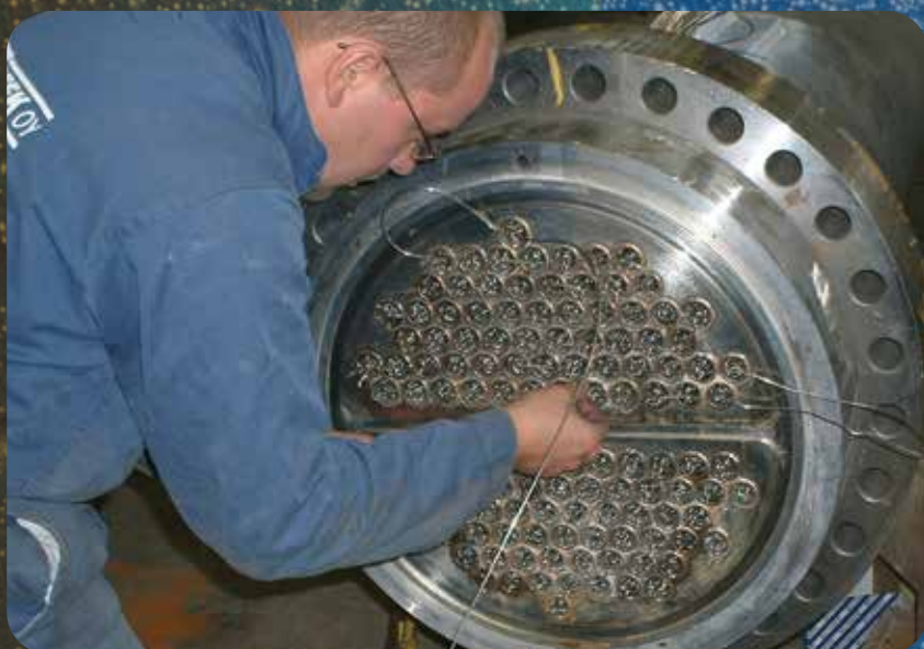
hiTRAN installation. Courtesy: KCC
