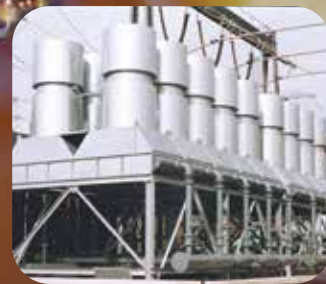
Transformer oil coolers. Courtesy: Spiro Gills, UK (GEA)
