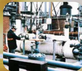
Ethylene let-down preheater. Retrofit to increase duty. Unit operating at critical temperature and pressure. Courtesy: European Vinyls Corporation
