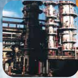
Stabiliser reboiler on crude unit. Installed: 1996. Location: Grangemouth, Scotland Courtesy: BP Oil, UK
