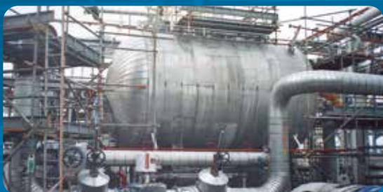
Ethylene vapouriser, Malaysia. Courtesy: Optimal Chemicals
