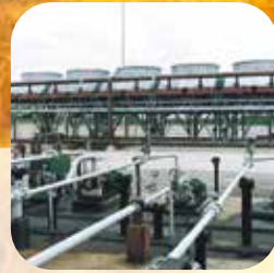
Gas oil run-down coolers. Location: Stanlow Refinery, UK Courtesy: Shell Oil, UK
